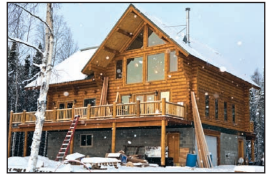
The Elkhorn 3,200-square-foot custom log home's four heating zones and four bathrooms are no strain for the Baxi boiler with Modulo tank.
